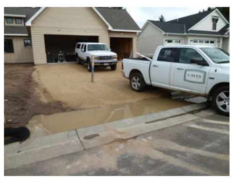
Access must be maintained to the very end of all construction
