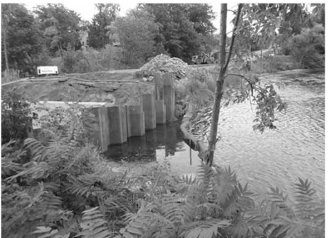
Sheeting holding out downstream water
