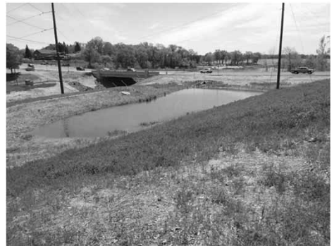
Nearing completion Pond cleaned out again and stabilized
