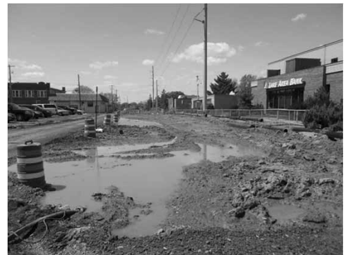
Solving storm water problems
