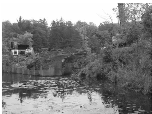
Tearing out old structure
