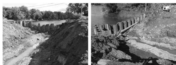
Old structure removed Down in the trench
