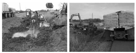
Directional drilling Know the material being used
