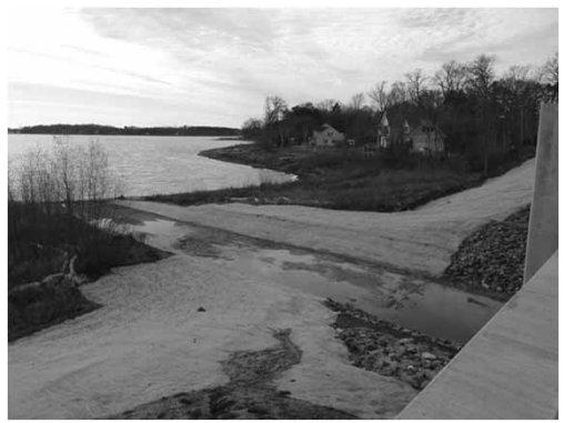
Stabilized for Fall
