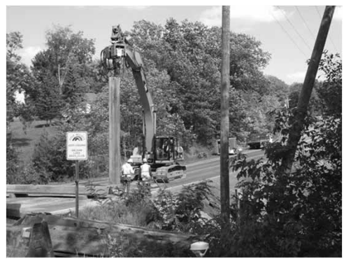
Starting the project... sheeting
