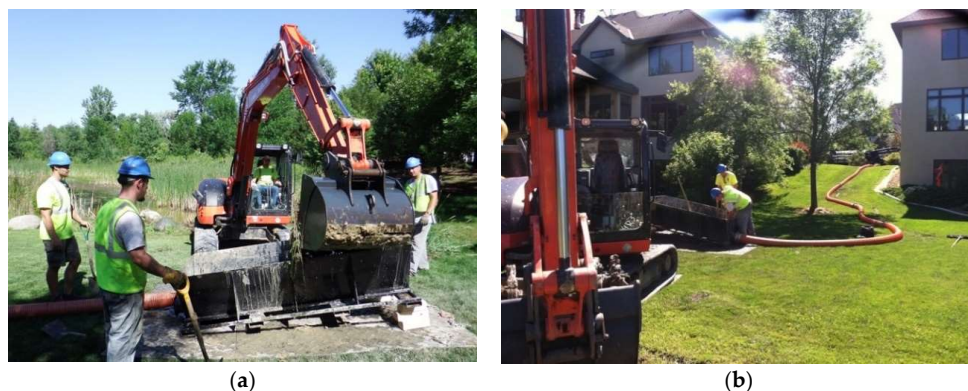
Figure 2. Dredged sediment being deposited into a vacuum dredge box (a) and vacuumed away to a truck on the street (b). Photos copyright of the City of Eden Prairie, MN, USA.
