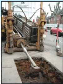
Drill Head and Launching Pit
